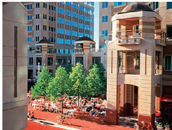
Architecture and landscape can also support the sense of arrival within a district.
